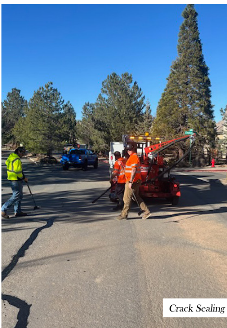
Crack Sealing
