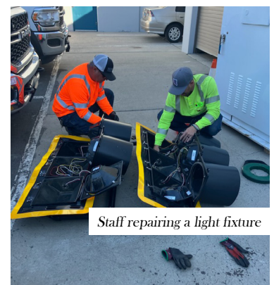
Staff repairing a light fixture
